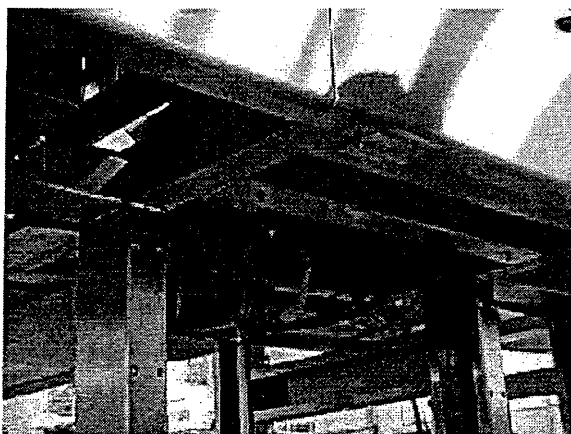
3. Condition with bottom cover removed.
