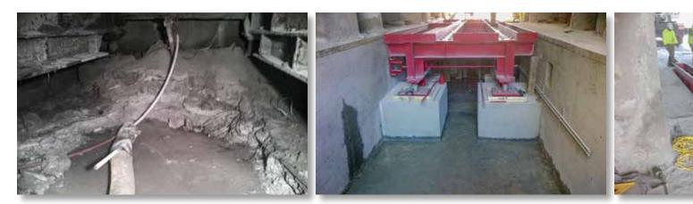
Photos by Brad Locker. After a thorough cleaning of the 50-year-old pit, Rice Lake's custom rail scale was expertly lowered into position and installed.
