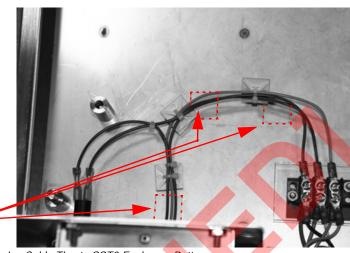
Figure 5-14. Secure Square Adhesive Cable Ties to SST3 Enclosure Bottom
