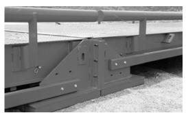
Figure 2-4. Two Self-Contained Module Connection (No Bridge Module)
