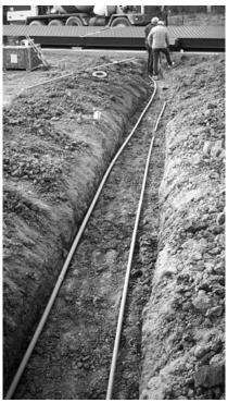
Figure 3-1. Conduit Run in Trench
