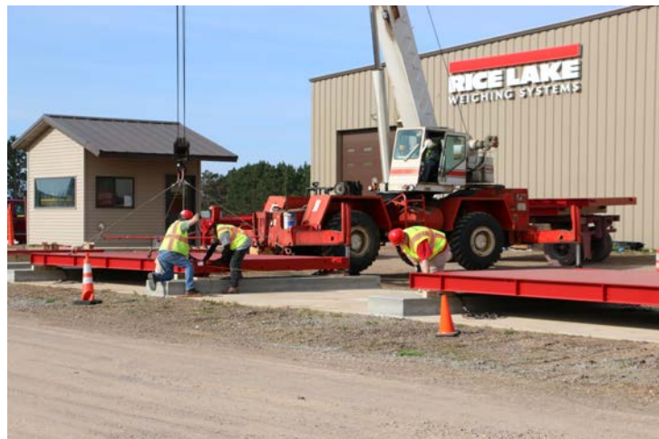
Figure 3-4. Setting Modules in Place
