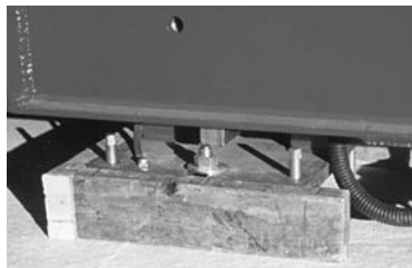
Figure 4-12. Temporary Wooden Forms Around Baseplate
