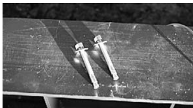
Figure 4-9. Anchor Bolts with Washers
