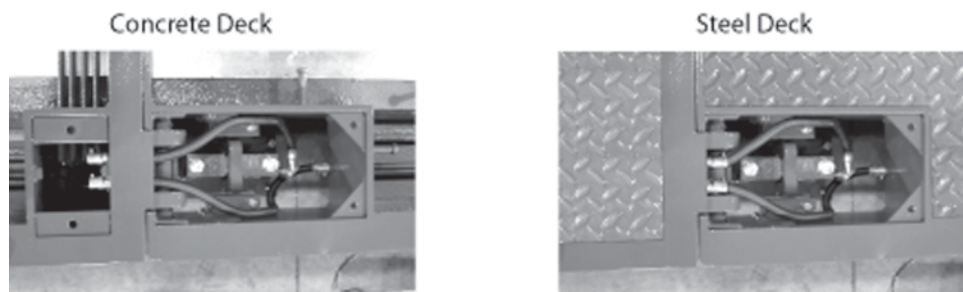
Figure 5-5. Conduit Connection Between Deck Modules
