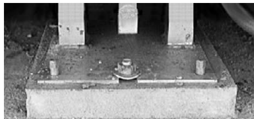
Figure 4-13. Completed Baseplate Grouting
