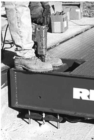
Figure 4-8. Drill Anchor Bolt Holes
