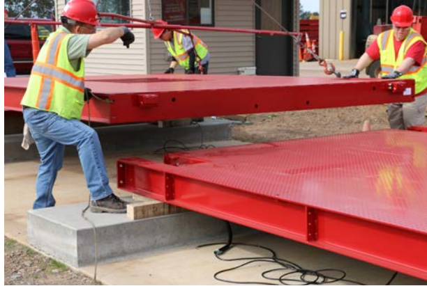
Figure 3-5. Module B Installation
