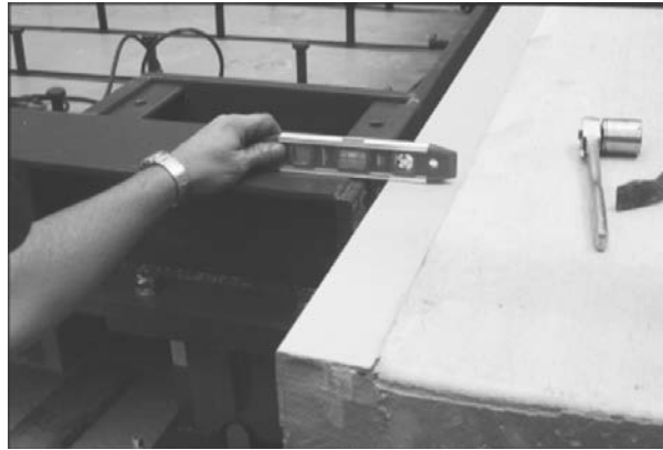
Figure 3-7. Leveling Deck with Approaches
