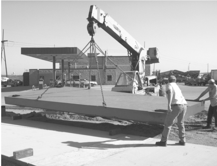
Figure 2-1. Lifting Deck Modules
