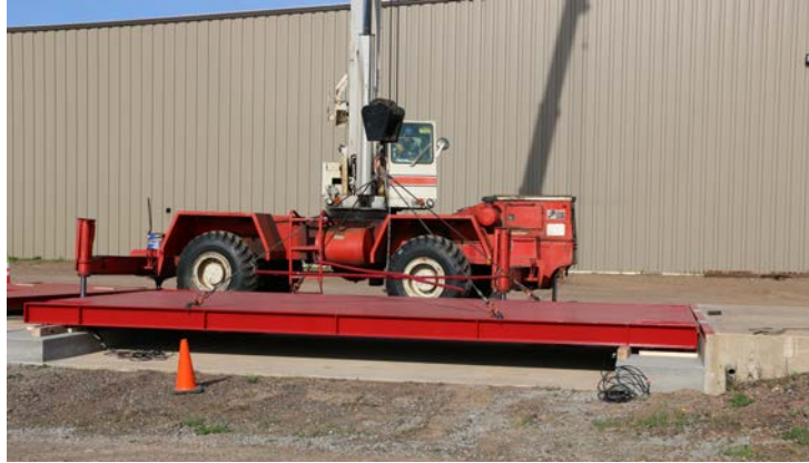
Figure 3-3. Module Positioned on Temporary Setting Blocks
