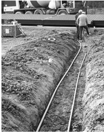
Figure 7-1. Conduit Run in Trench
