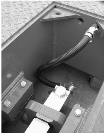
Figure 5-3. Load Cell Pocket Conduit Installed
