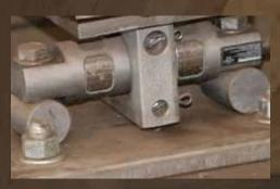
FM-approved load cells are installed under the distillery's 6,000+ gallon, stainless steel storage tanks.
