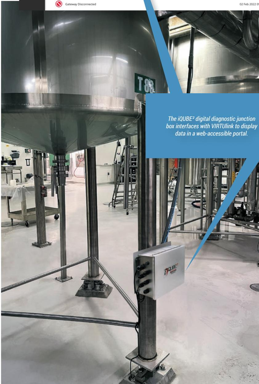
The iQUBE<sup>2</sup> digital diagnostic junction box interfaces with VIRTUlink to display data in a web-accessible portal.
