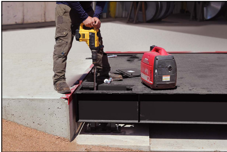
Figure 3-13. Drill Anchor Bolt Holes
