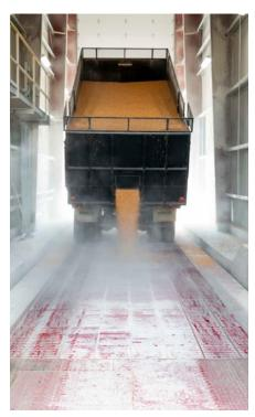
Grain dump grating is an option for many truck scale models but consulting with an expert can ensure you find the best solution for your facility.
