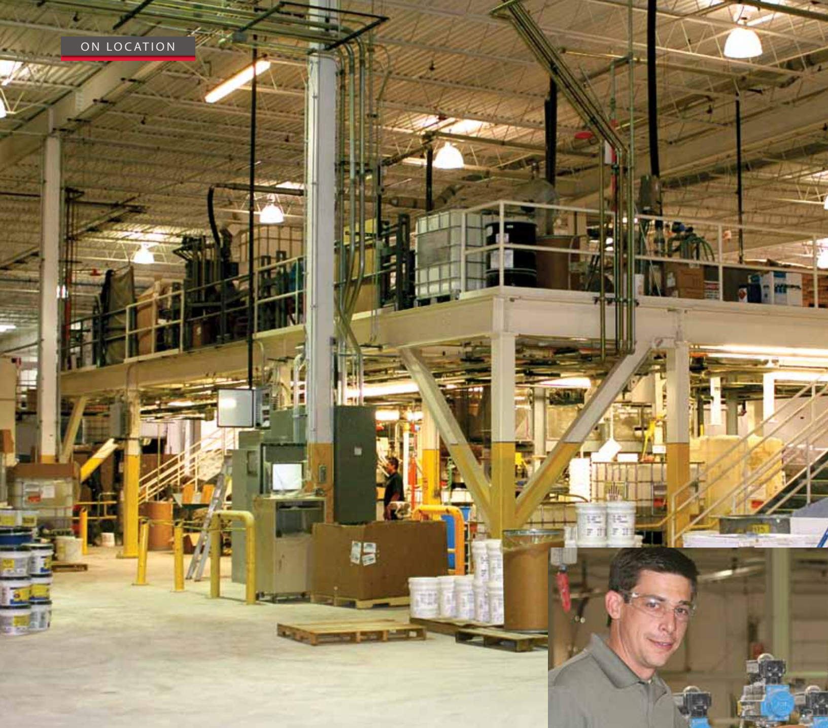
H.B. Fuller Construction Products built a mezzanine to accommodate a variety of new processing and packaging equipment being moved from another facility. They were tasked to combine the new equipment into the existing manufacturing area and be up and running in 90 days.
