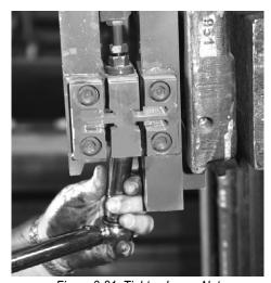
Figure 3-21. Tighten Lower Nut
