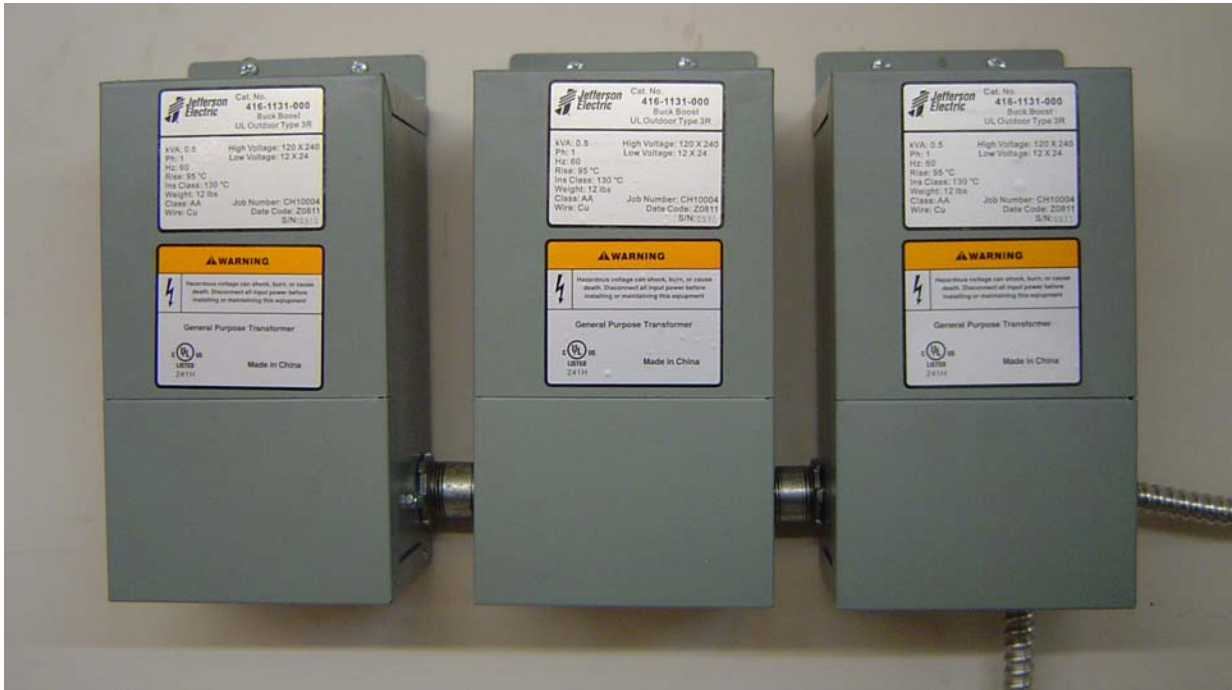
Figure 5. Three Buck-Boost Transformers for 3-Phase Wye Configuration
