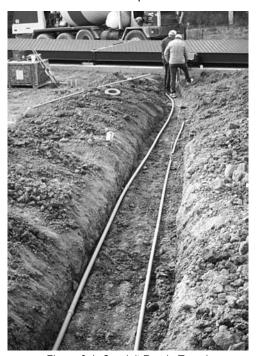
Figure 6-1. Conduit Run in Trench
