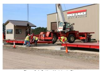
Figure 3-4. Setting Modules in Place
