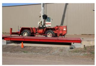
Figure 3-3. Module Positioned on Temporary Setting Blocks
