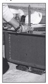
Figure 4-10. Seating Anchor Bolts on Baseplate
