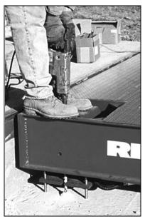
Figure 4-8. Drill Anchor Bolt Holes
