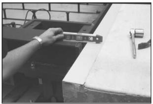
Figure 3-7. Leveling Deck with Approaches
