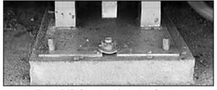
Figure 4-13. Completed Baseplate Grouting
