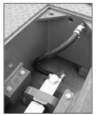
Figure 5-3. Load Cell Pocket Conduit Installed
