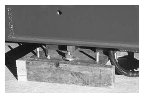
Figure 4-12. Temporary Wooden Forms Around Baseplate
