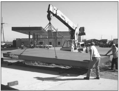
Figure 2-1. Lifting Deck Modules
