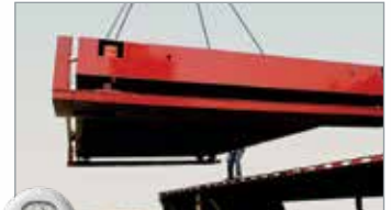
2 Unload modules on level, solid ground.
