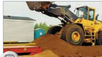
3 Backfill to bulkheads and finish ramps.
