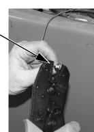
Figure 3-5. Attach Terminals to Power Cable - Battery End
