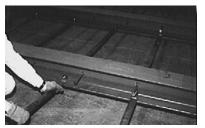
Unload the support bars from the hardware box on the truck. Each group of similar-length bars is bundled separately and marked. Keep equal length bars together in separate piles.
