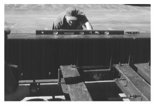
When the entire deck frame is level, torque down all cross beam bolts to 260 ft. lb.
