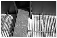
Cut out clearance sections in the panels for drain tubes where necessary. Slide the main panel into place, then make a larger overlapping panel section with a slot cut out for the drain tube. Slide the overlapping panel into place aligned with corrugations of the main panel. Use duct tape to seal the panel for the concrete deck pour
