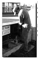
Use an industrial hammer drill with a 3/4" carbide masonry bit at least 36" long to drill anchor bolt holes. This long bit allows the drill body to clear the siderail so the hole can be drilled nearly vertical. Hold the bit as close to vertical as possible and drill a 3/4" hole at least 6" into the concrete beneath each anchor bolt slot on both sides of the baseplate.
