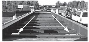
Move down the scale toward the other end, jacking and shimming until the entire deck is level in both directions.
