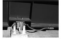
All areas of cabling where rigid conduit might affect load cell deflection must use flexible cable sections. This includes cable sections adjacent to load cells as in the photo at left. In this application, a threaded LB fitting connects the flexible section to the rigid conduit running beneath the scale deck to the junction box on the opposite siderail.
