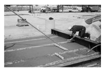
Continue with each section in the same manner. As a general guideline, a 90' x 14' deck 8" thick should require approximately 30-32 cubic yards of concrete, necessitating two or possibly three concrete trucks. A short break between trucks will allow time to finish float and edge poured sections while waiting for the next concrete truck. Don't forget to clean out concrete from the drain tubes on each bay.
