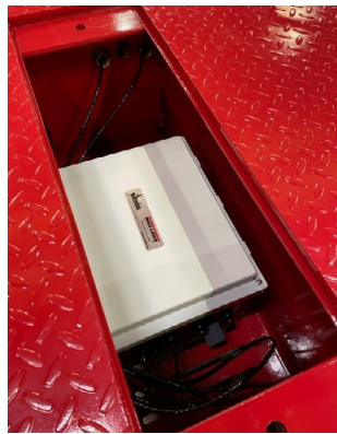
Figure 5-4. Junction Box Pocket
