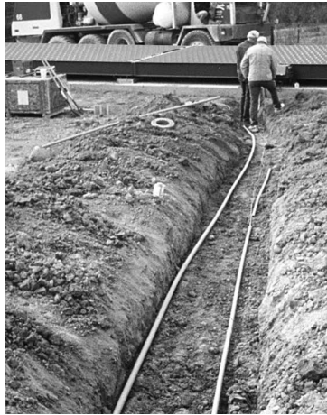
Figure 7-1. Conduit Run in Trench
