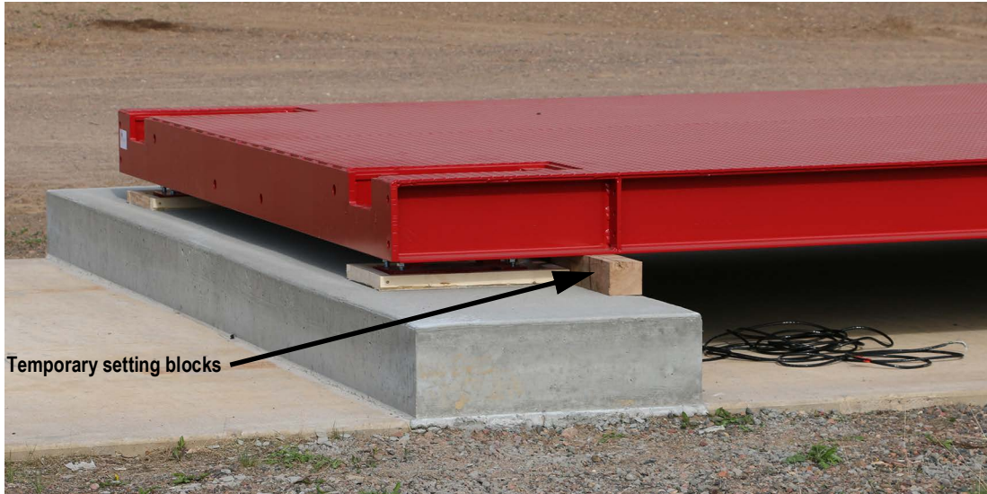
Figure 3-3. Module Positioned on Temporary Setting Blocks
