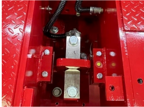
Figure 5-3. Load Cell Pocket Conduit Installed
