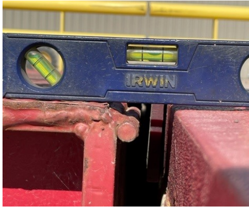
Figure 3-7. Leveling Deck with Approaches
