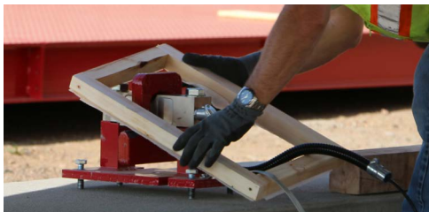
Figure 4-12. Temporary Wooden Forms Around Baseplate
