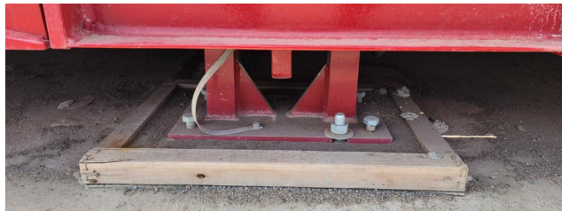
Figure 4-13. Framed and Grouted Baseplate
