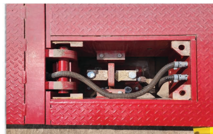
Figure 5-5. Conduit Connection Between Deck Modules
