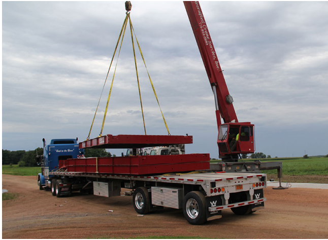
Figure 2-1. Lifting Deck Modules
