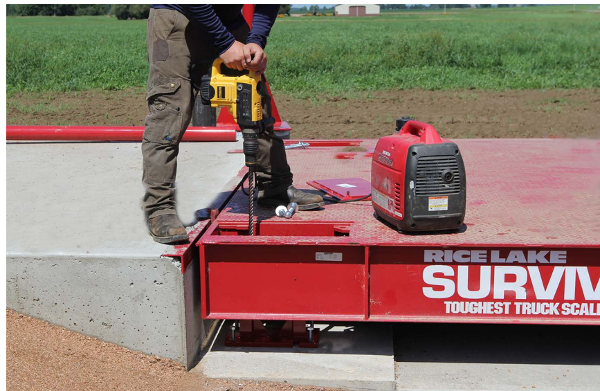
Figure 4-9. Drill Anchor Bolt Holes
