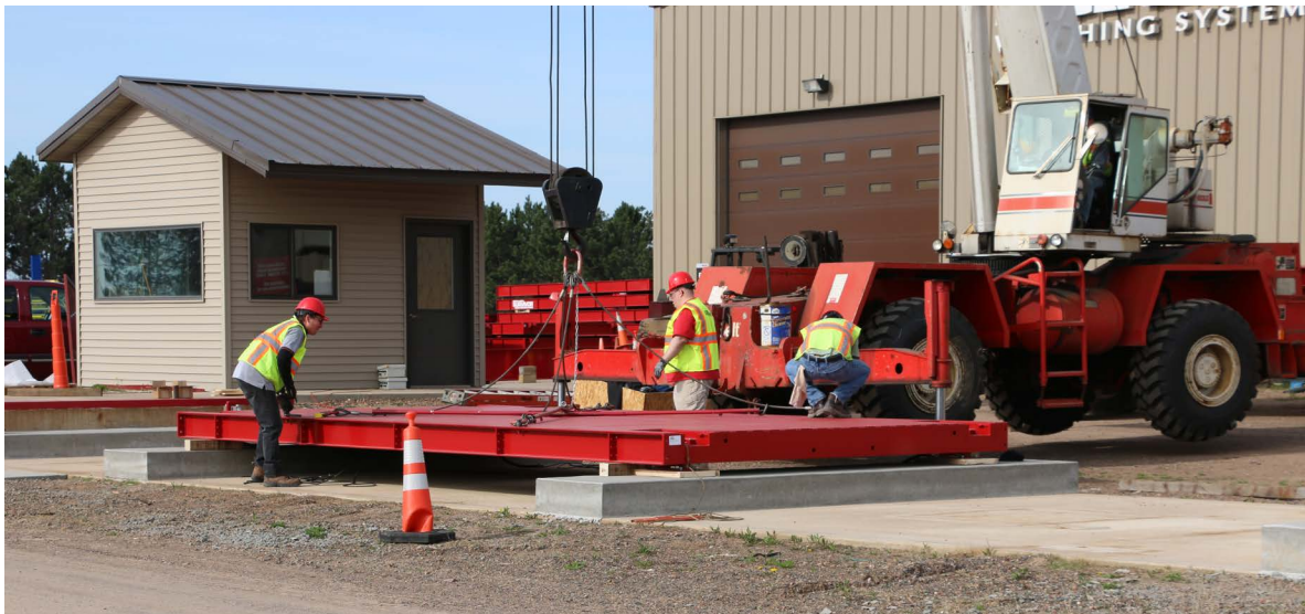
Figure 3-4. Setting Modules in Place
