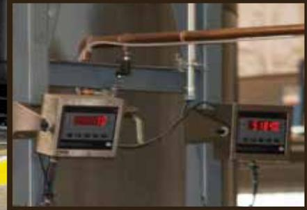
T4 temperature rating and Factory Mutual (FM) approval for hazardous environments. The indicator's power supply is intrinsically-safe and auto-ranging, allowing for simplified wiring to a single AC conduit line and seal from a safe area. The
