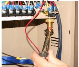
12. Loosen but do not remove the top valve fitting by using an adjustable wrench.
