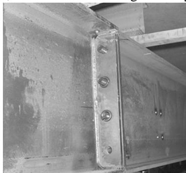
Figure 2-2. Top Bolts, Washers, and Nuts Installed
