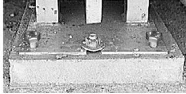
Figure 3-7. Grout example.
