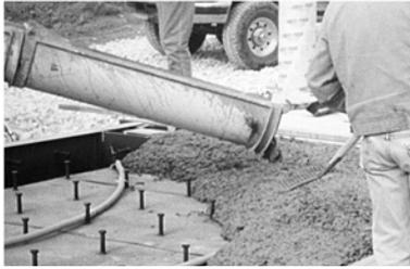
Position the unloading chute at the near left side of the scale and begin filling having the truck move slowly to the right.
