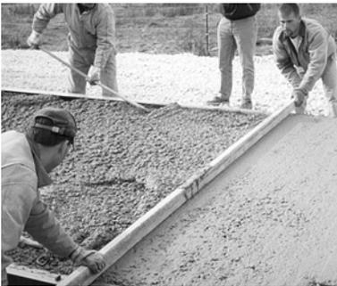
After vibrating to approximate level, screed the concrete to the level of the top of the support channels with a 2x4 board cut to length
