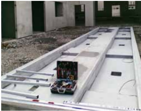
Example of a new installation
