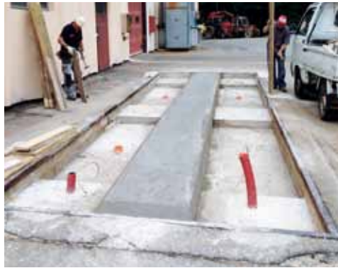
Example of a recycled existing pit
