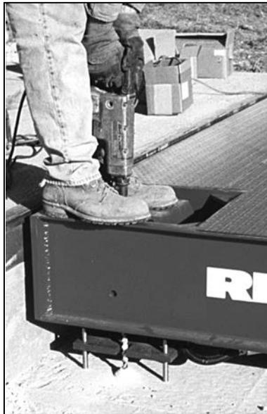
Figure 4-8. Drill Anchor Bolt Holes
