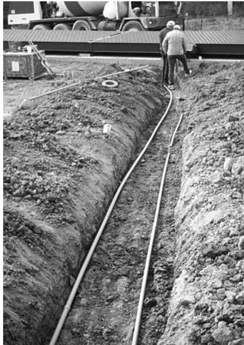
Figure 6-1. Conduit Run in Trench
