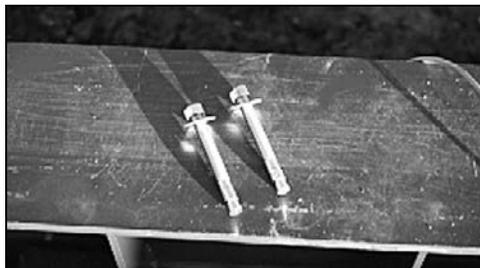
Figure 4-9. Anchor Bolts with Washers
