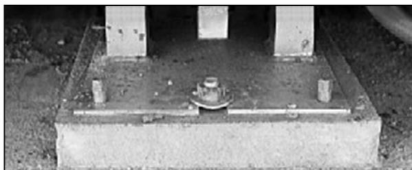
Figure 4-13. Completed Baseplate Grouting
