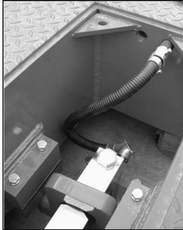
Figure 5-3. Load Cell Pocket Conduit Installed
