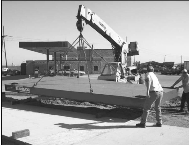
Figure 2-1. Lifting Deck Modules
