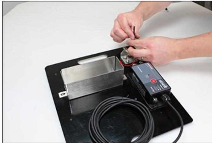
Figure 2-4. Antenna Bracket Mount Installation
