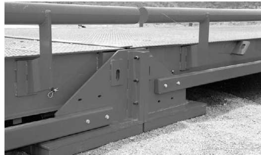
Figure 2-4. Two Self-Contained Module Connection (No Bridge Module)
