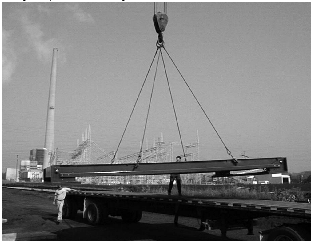
Figure 1-2. Unloading Modules From Truck
