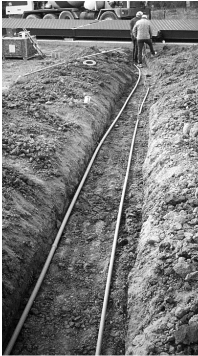
Figure 3-1. Conduit Run in Trench
