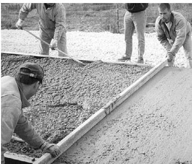
Figure 4-4. Screeding Concrete
