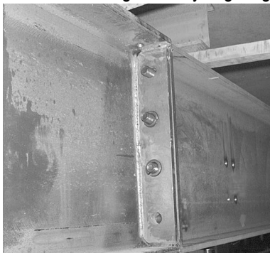
Figure 2-2. Top Bolts, Washers, and Nuts Installed
