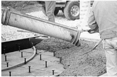
Figure 4-2. Filling Concrete
