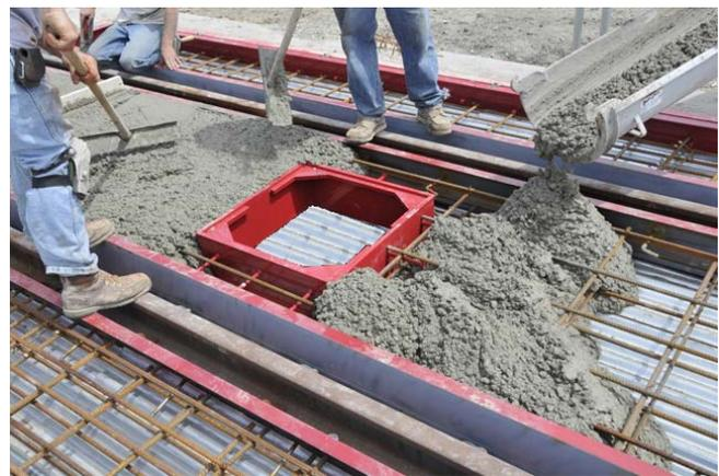
Figure 2-19. Rebar Installed (Left) and Pouring Concrete (Right)
