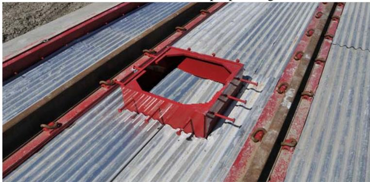
Figure 2-18. Manhole Frame
