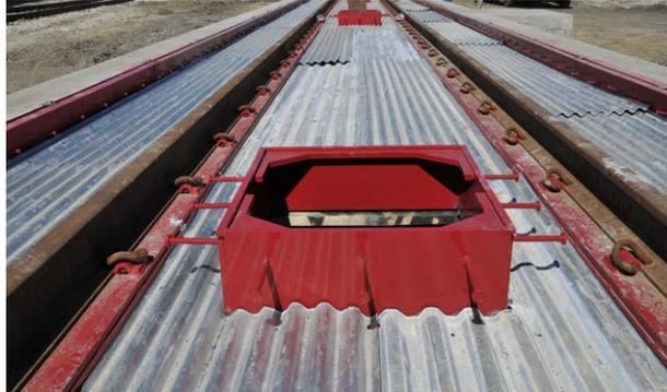
Figure 2-17. Deck Pan Installed
