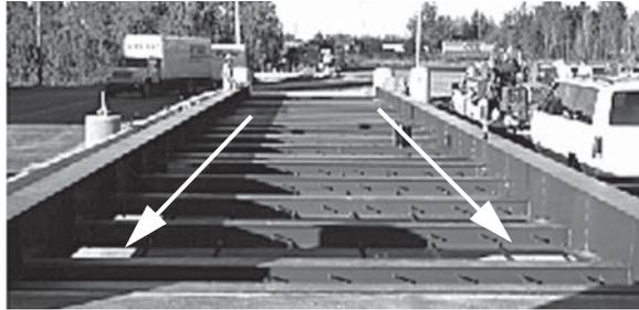
Move down the scale toward the other end, jacking and shimming until the entire deck is level in both directions.
