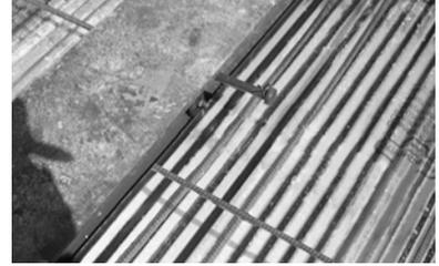
Tie rebar parallel to the siderails under the Nelson studs on each siderail. Using these rebars along the siderails for support, set and tie long rebars each 8" parallel to the cross beams.
