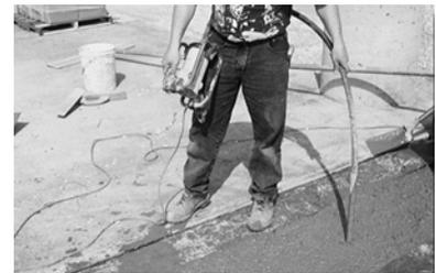
After vibrating to approximate level, screed the concrete to the level of the cross beams with a 2x4 board cut to the appropriate length. As this first bay is too narrow to use a wide bull float, the final surface leveling should be done with a magnesium hand float.
