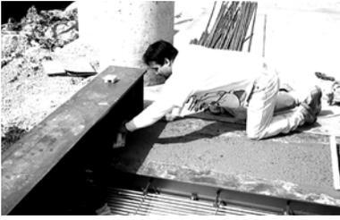
With the bay level and floated, finish against the siderails with either a magnesium float or steel trowel for a neat deck line level with the exposed cross beams. If you have taped plastic-film splatter guards on the siderails, the bottom tape strip will serve as a guide for the finished deck level between cross beams.
