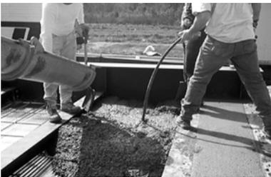
Move to the next section and pour and vibrate that section.
