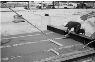
Continue with each section in the same manner. As a general guideline, a 90' x 14' deck 8" thick should require approximately 30-32 cubic yards of concrete, necessitating two or possibly three concrete trucks. A short break between trucks will allow time to finish float and edge poured sections while waiting for the next concrete truck. Don't forget to clean out concrete from the drain tubes on each bay.
