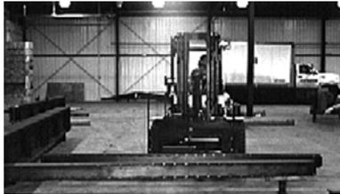
Bring the cross beams onto the pad one at a time starting at one approach end. Position each cross beam at its final location with one end resting on the side rail flange. Bolt the cross beam to the side rail. Rest the other end of the cross beam at a right angle to the side rail on a setting block 2" higher than your 8" blocks. Repeat for all cross beams of the module.
