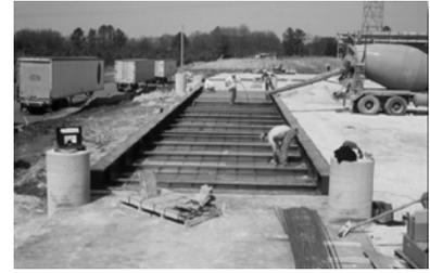
To protect against unsightly concrete splatters on the inside of the siderail beams, you may want to tape 4-6 mil plastic against the inside surface of the siderails starting at the finished deck level (top of cross beams) and running up the siderail several inches. If applied carefully, the bottom tape strip can serve as a screed guide for the concrete deck surface against the siderails.
