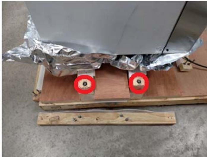
4.3 Using a **30mm** wrench (or **1.25"** adjustable) lower all **four** leveling feet, in even increments, until the wrapper just clears the 4x4 bracing then remove the bracing:
