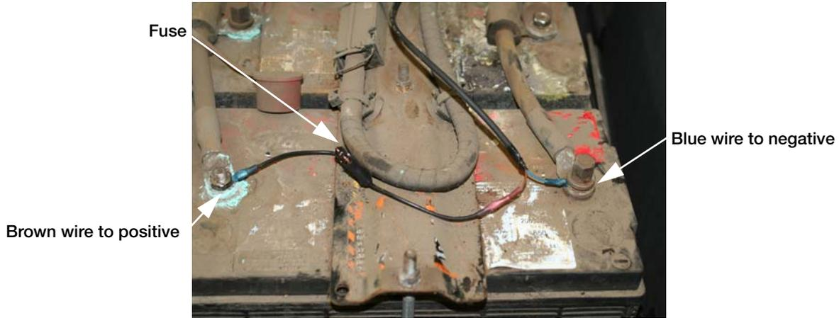
Figure 3-5. Power Connection to Battery
